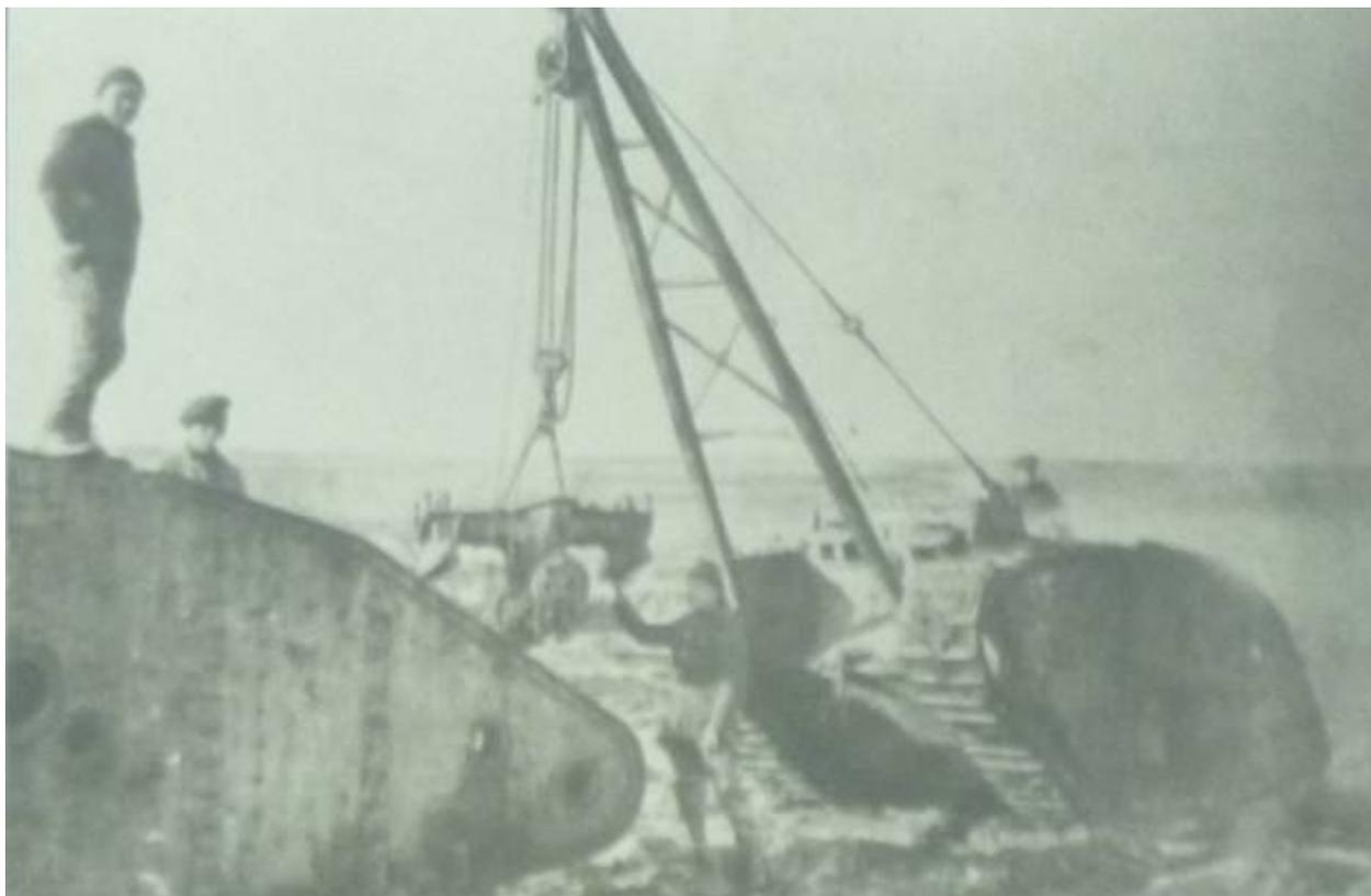
The picture on the previous page shows a small section of men from a Salvage Company, it appears, removing part of the transmission to the rear geared wheels. Whether the tank was damaged elsewhere or not, it is difficult to say, but it may not have been capable of moving under tow, say, with its transmission jammed. A tank such as that on the right, fitted with the jib and block and tackle would have easily supported a sponson during its fitment or removal.
