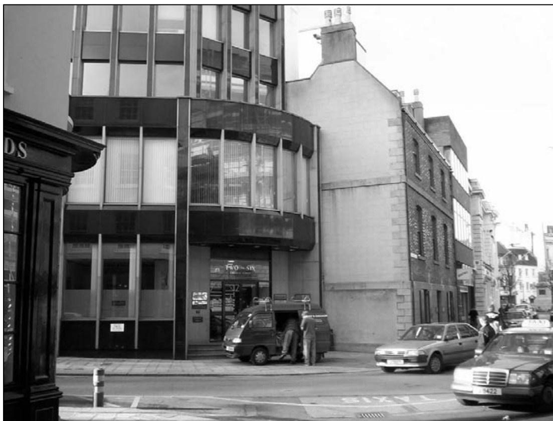
The site of the former French Consulate in St Helier’s Church Street
